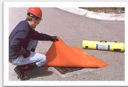
Protect the storm drain
